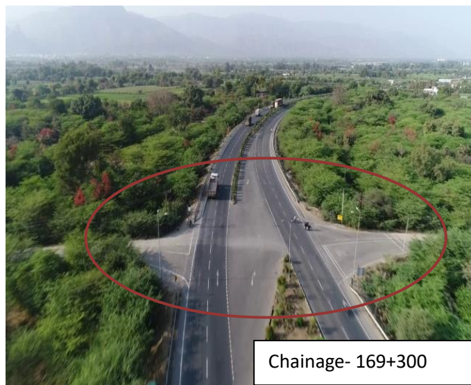
Figure 5.1: Deficiencies in Minor Junction along the Study Stretch
