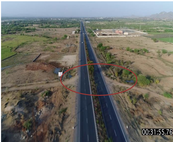
Figure 5.2: Unauthorized Ramps along the Study Stretch
